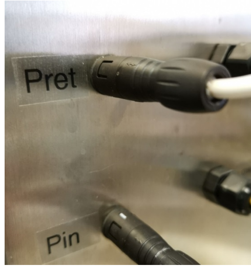
Sample installation with 2 sensors connected
